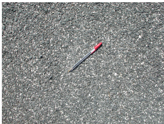
Figure 3. Example of an asphalt pavement of the study area with surfacing limestone granules.
