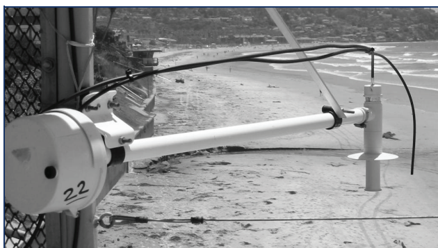
Fig. 3. Photo showing the setup of the two-intake test.
